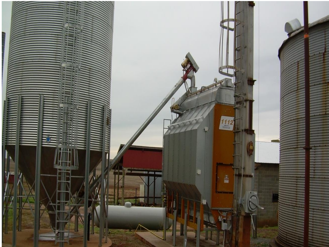
Grain Dryer Replacement Brandy Station, VA
