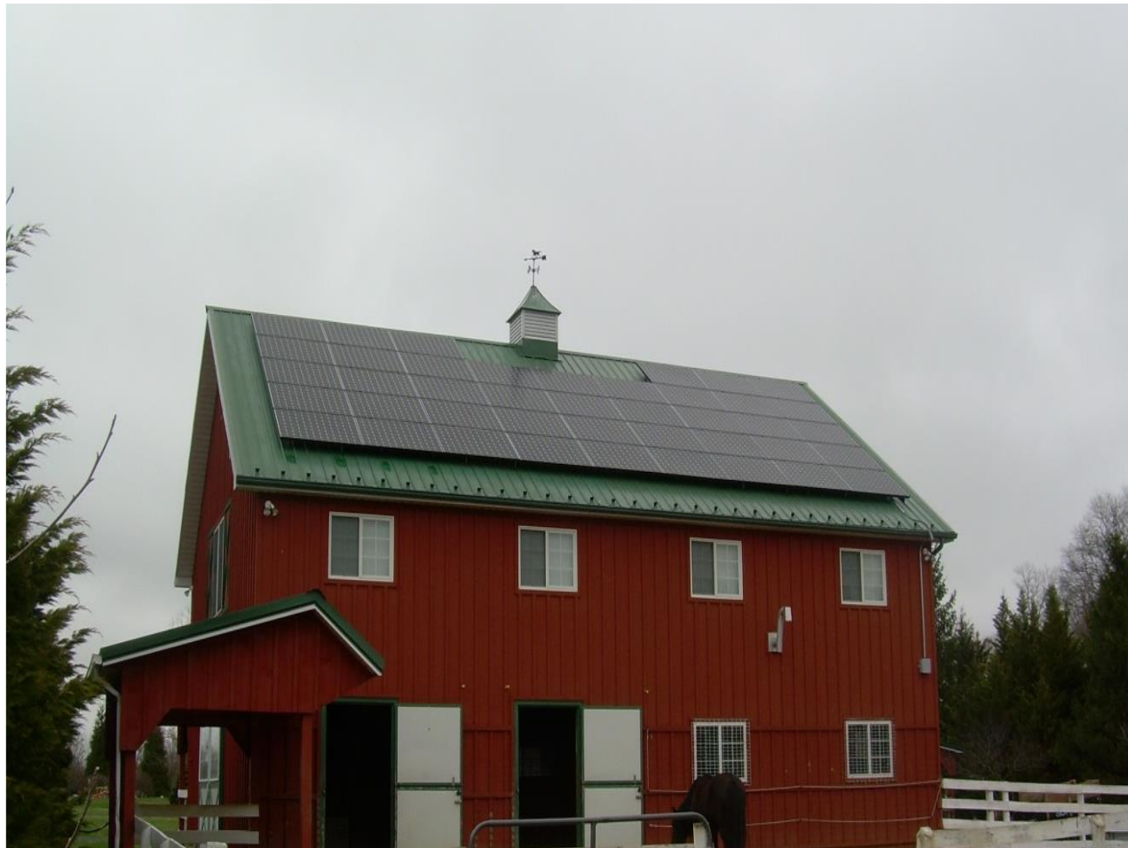
12.4 kW Roof-Mounted Solar Purcellville, VA
