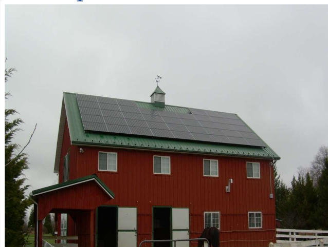
12.4 kW Roof-Mounted Solar Purcellville, VA
