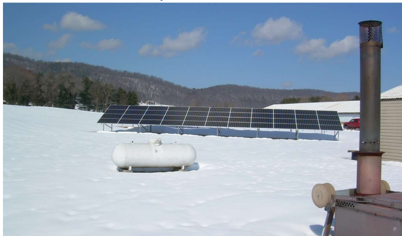
40 kW Ground-Mounted Solar Mount Crawford, VA
