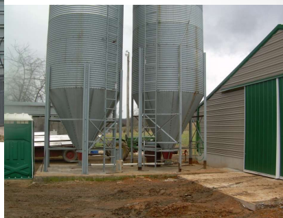
Poultry House Replacement Mount Solon, VA
