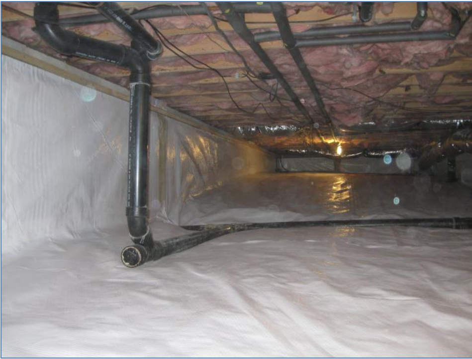
Photo: 37: A view of the poly-liner and furring strip holding it up before insulation is installed;
