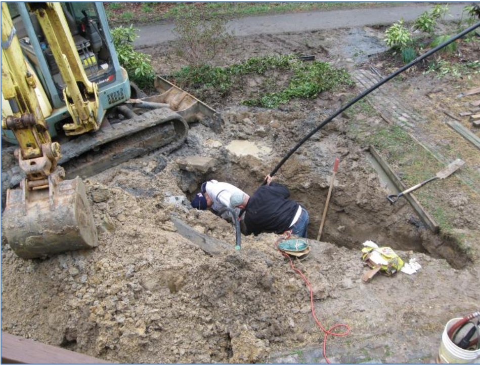
Photo: 22: Thermally fusing a connecting piece onto the vertical loop
