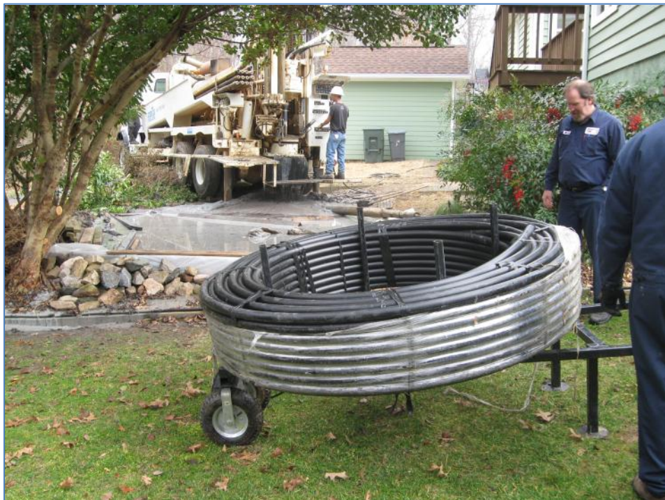
Photo: 14: Another view of the geo-loop, all 500+ ft. of it ready to be inserted down the boring;
