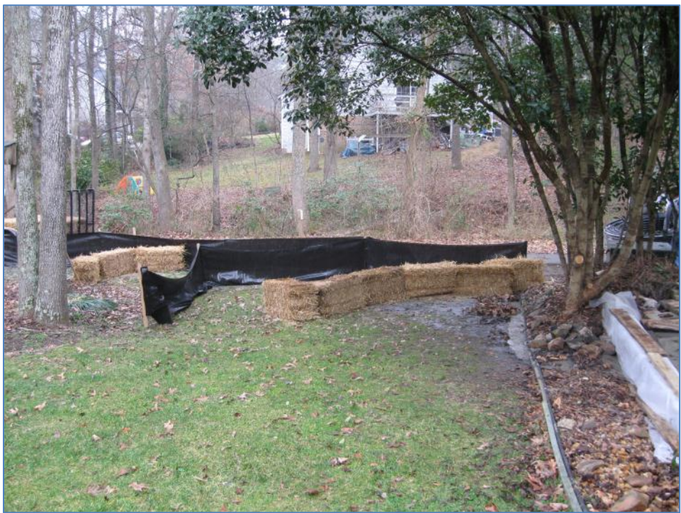
Photo: 11: Bales of straw and silt-fencing placed to capture run-off from the site;
