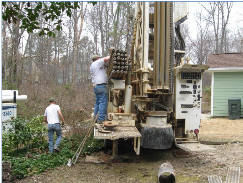
Photo 5: Drill rig preparations; the operator is picking up the first 20ft. section of drilling pipe;
