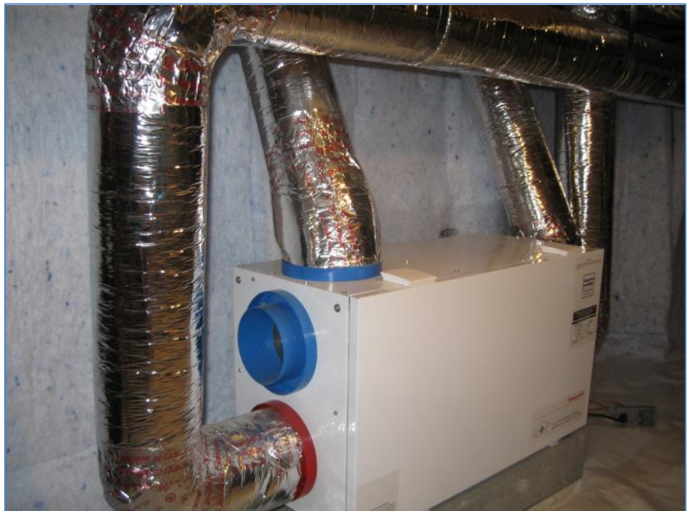
Photo: 34: Close-up of the Honeywell Energy Recovery Ventilator (ERV);
