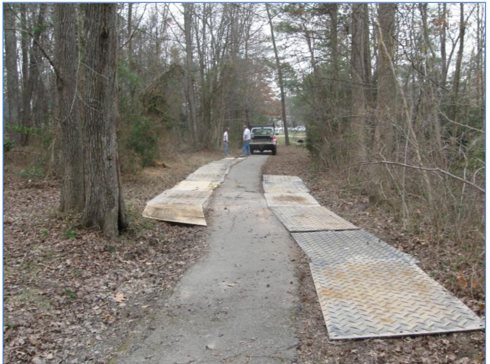
Photo 2: More steel sheeting and plywood laid in place before the drill rig accesses the trail/ common property;
