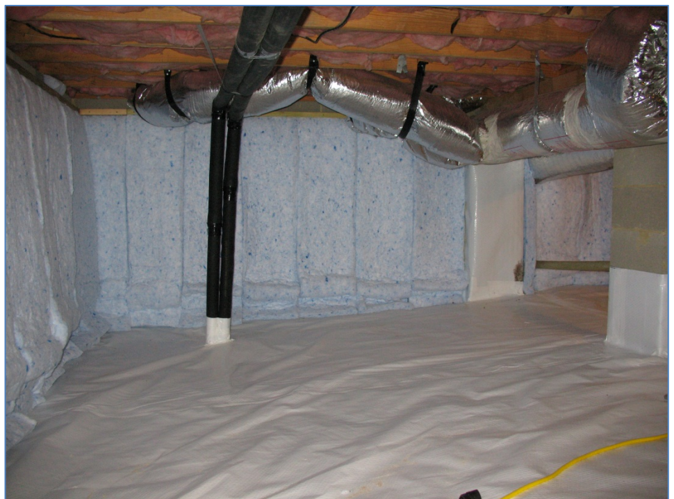
Photo: 40: Another view of the encapsulation and insulation job my oldest son and I did; note the geo-loop lines (in and out) that emerge from the crawl space floor and run along the floor joists;
