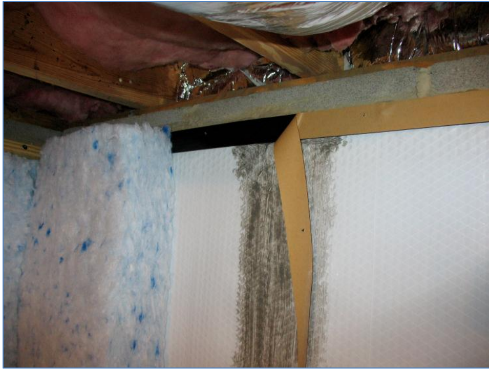
Photo: 35: Close-up of encapsulation with insulation; note 3" space of viewable foundation wall for termite inspection, black mastic sealant over poly-liner joint and 2-sided butyl rubber tape used to hold insulation until a 2 nd furring strip can be installed to permanently hold insulation;
