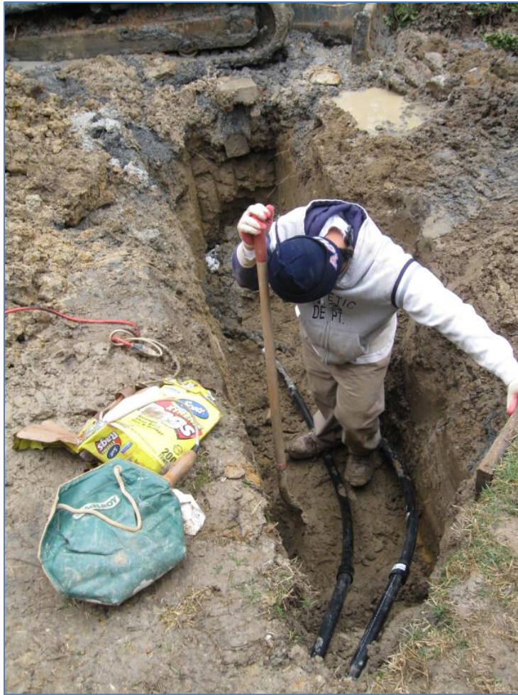
Photo: 24: Fusing complete; now to fill the trench with soil;
