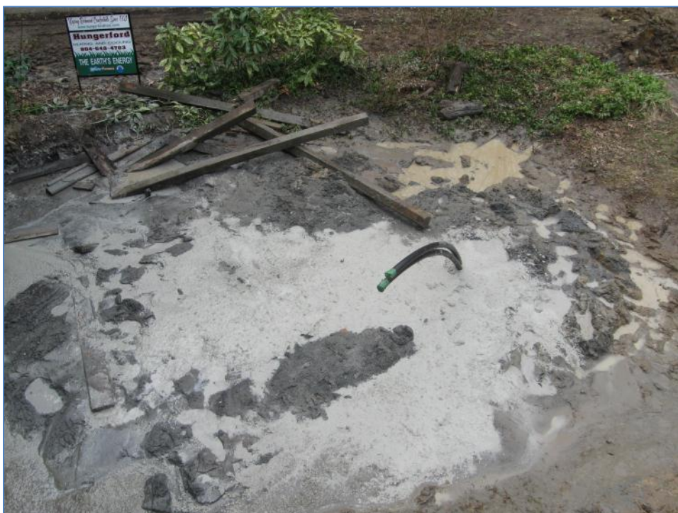
Photo: 20: Drill site after completion with the loop sticking up with the ends taped off until it can be connected
