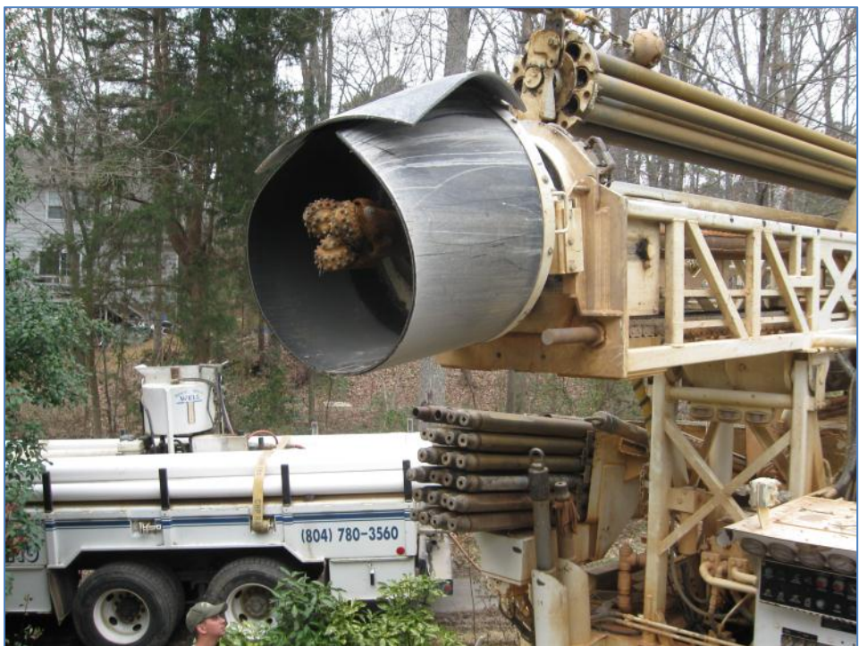
Photo 7: View of the rotary drill bit and a support truck loaded with 20ft. sections of PVC casing to line part of the boring;
