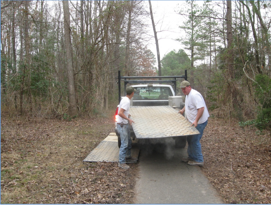
Photo 1: Drilling rig employees laying down steel sheets and plywood to guard against damage from the rig's weight/tires;
