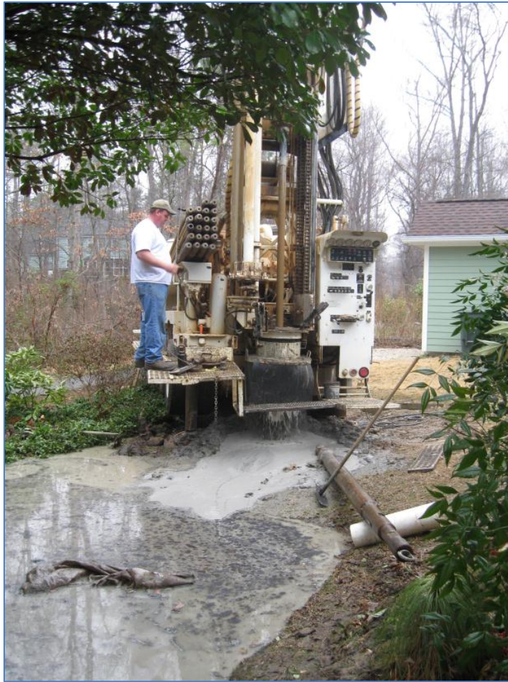
Photo: 13: Quite a lot of ground water came up during the drilling;
