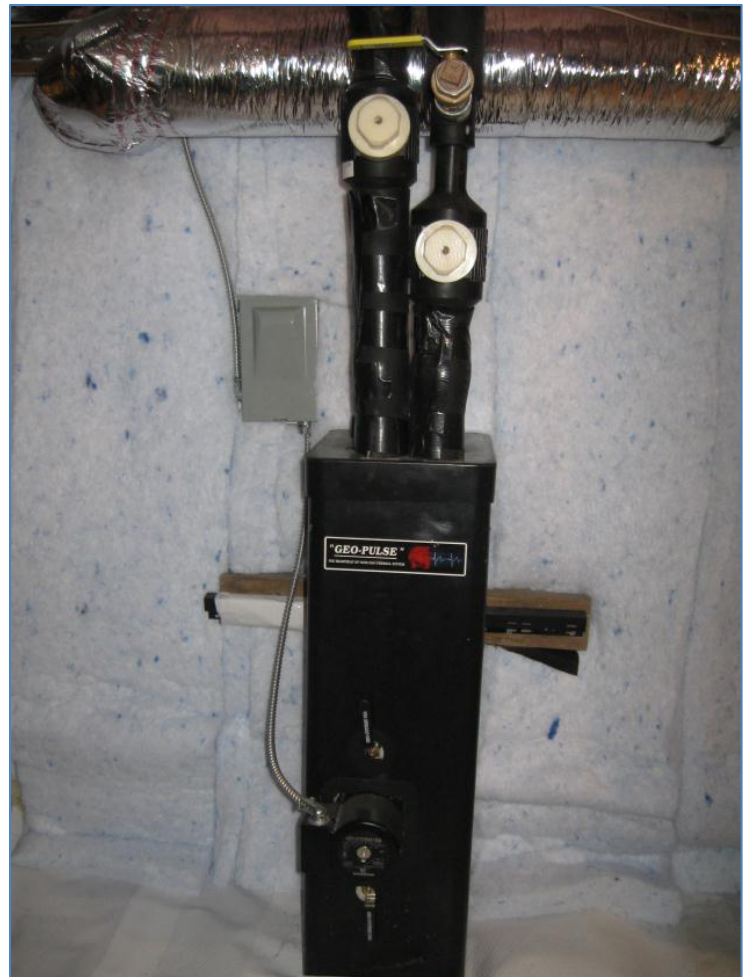
Photo: 32: And here is the "Geo-Pulse Flow Center" (fluid circulation pump);
