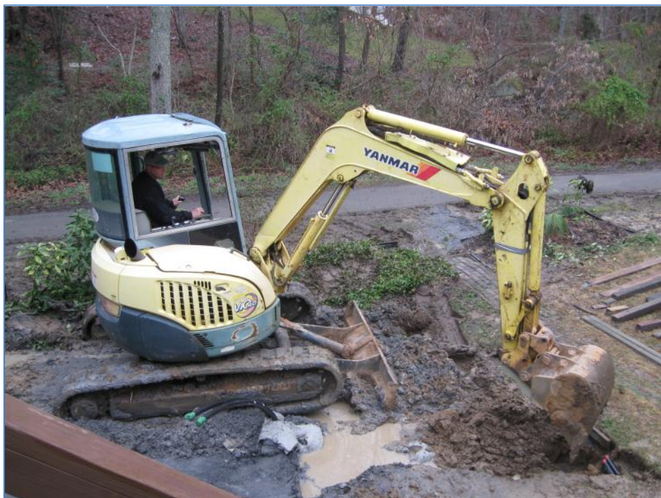
Photo: 21: Virginia Energy Services (sub-contractor) beginning to excavate so the vertical loop (green tape on ends) can be connected to the already installed section of pipe in the crawl space (red tape on ends in the lower right-hand corner);
