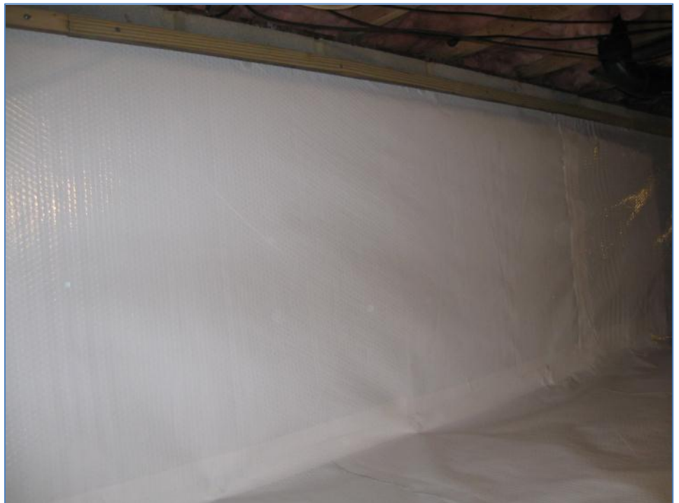
Photo: 38: A close-up of the same section of liner and furring strip before the insulation is hung; We used a 12mil polyethylene liner sourced from Americover, Inc.(see www.americover.com )
