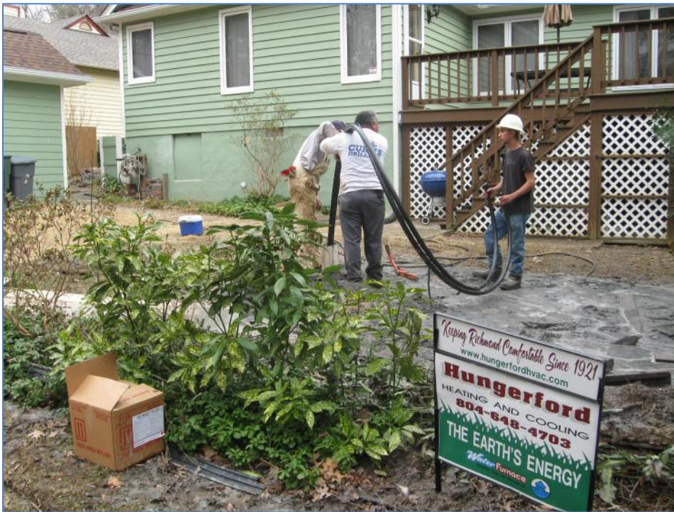
Photo: 18: Drilling crew inserting the last several feet of the geo-loop;
