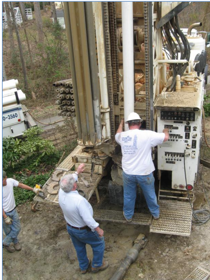
Photo: 10: The first 20ft. section of PVC casing being inserted down the boring;
