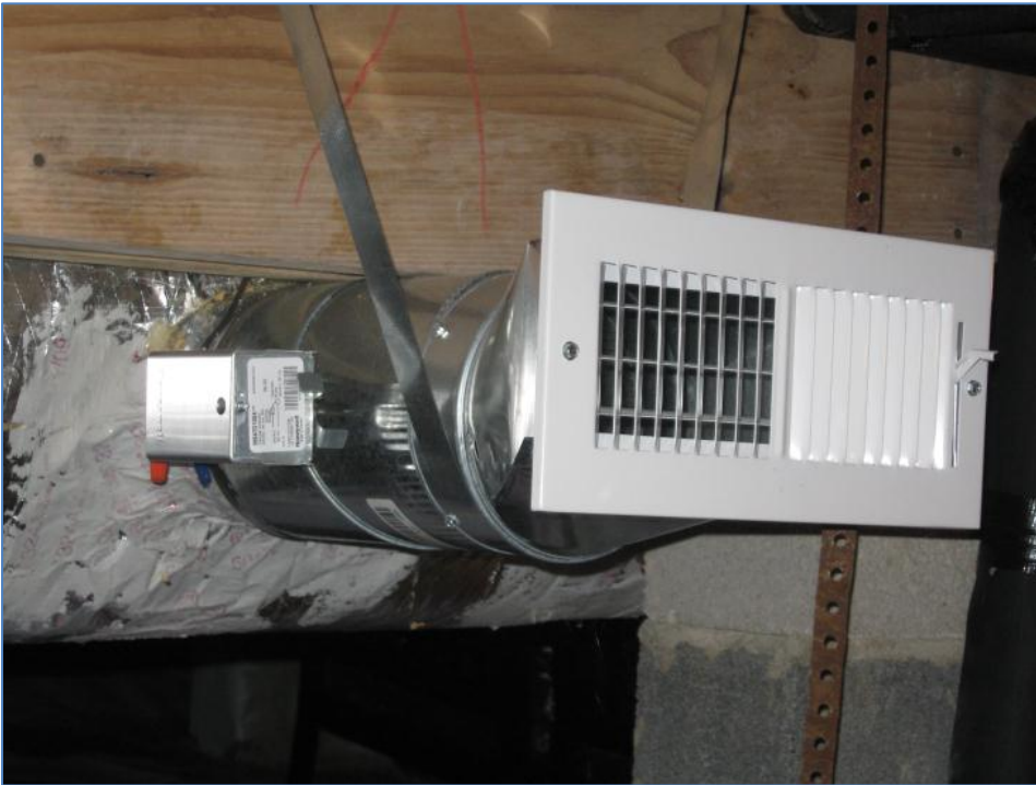
Photo: 33: Close-up of the dedicated vent in our crawl space; note actuator on the left-hand side that opens and closes the vent when the unit turns on and off;
