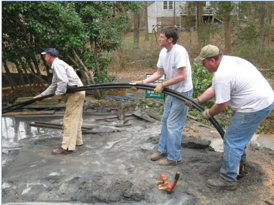
Photo: 17: Unrolling and shoving the loop into the boring;
