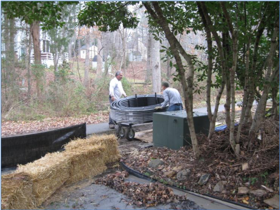
Photo: 12: Coiled-up 500ft. + long geo-loop rolled to the site;
