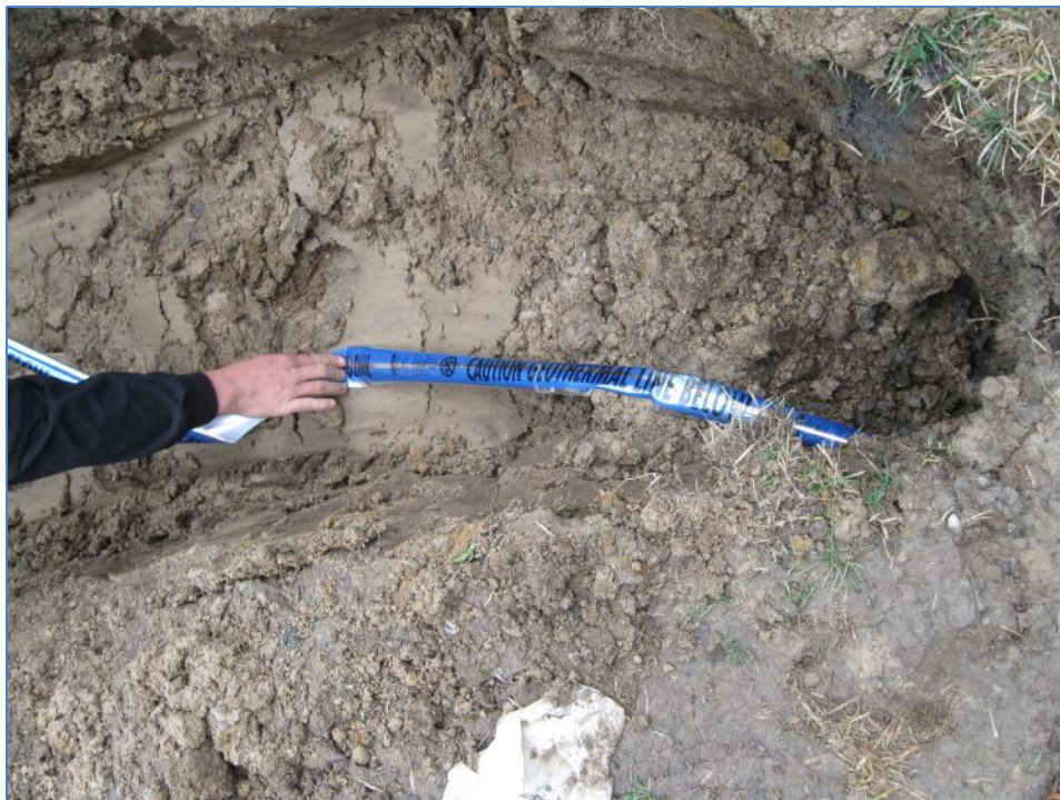
Photo: 25: Placing detectable magnetic tape over each line of loop so Miss Utility can find it if/when needed;
