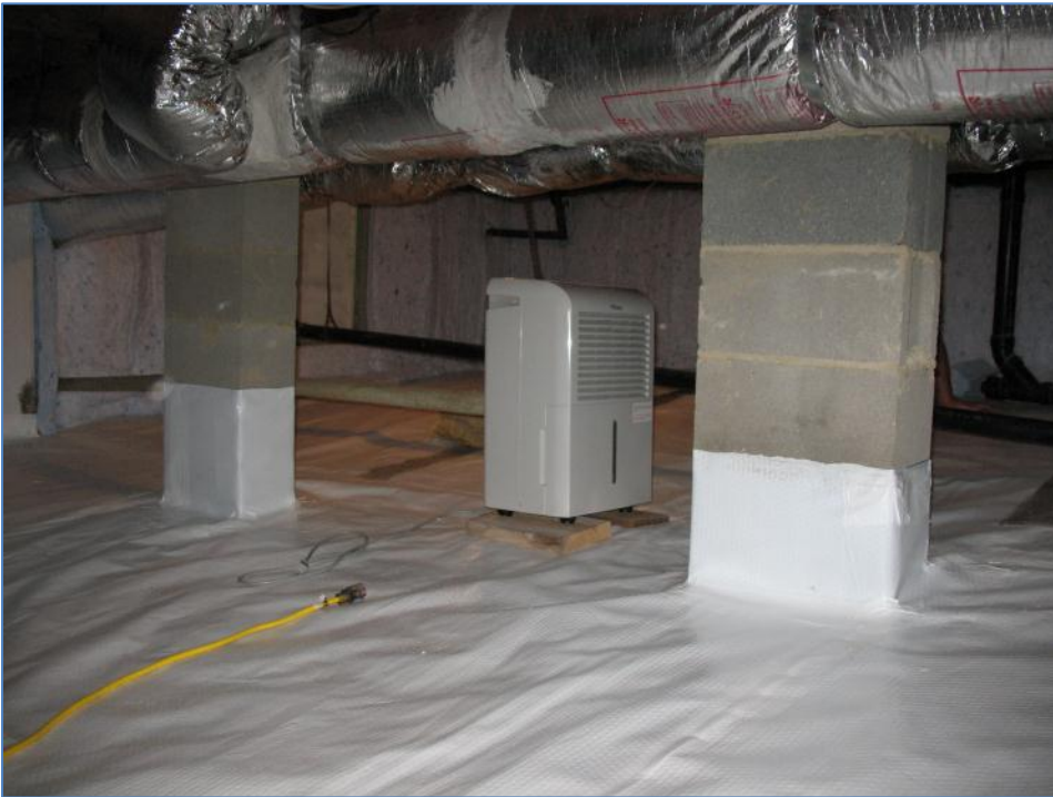
Photo: 39: A view of encapsulation of our crawl space with wrapped piers and insulated walls; also note the low-cost dehumidifier we bought and installed (condensation gravity feeds down PVC pipe that passes through the foundation wall where our old air-source unit's copper pipe used to pass;
