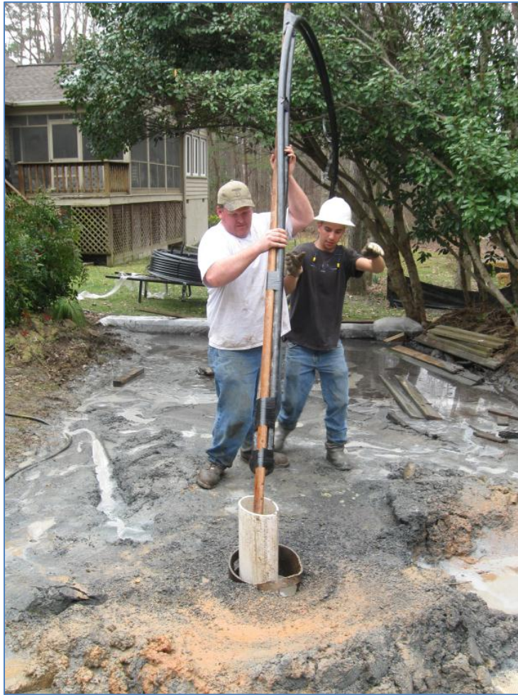
Photo: 16: The drilling crew inserting the “U-bend” formed end of the geo-loop into the boring (attached to a heavy piece of rebar to help pull the end to the bottom);
