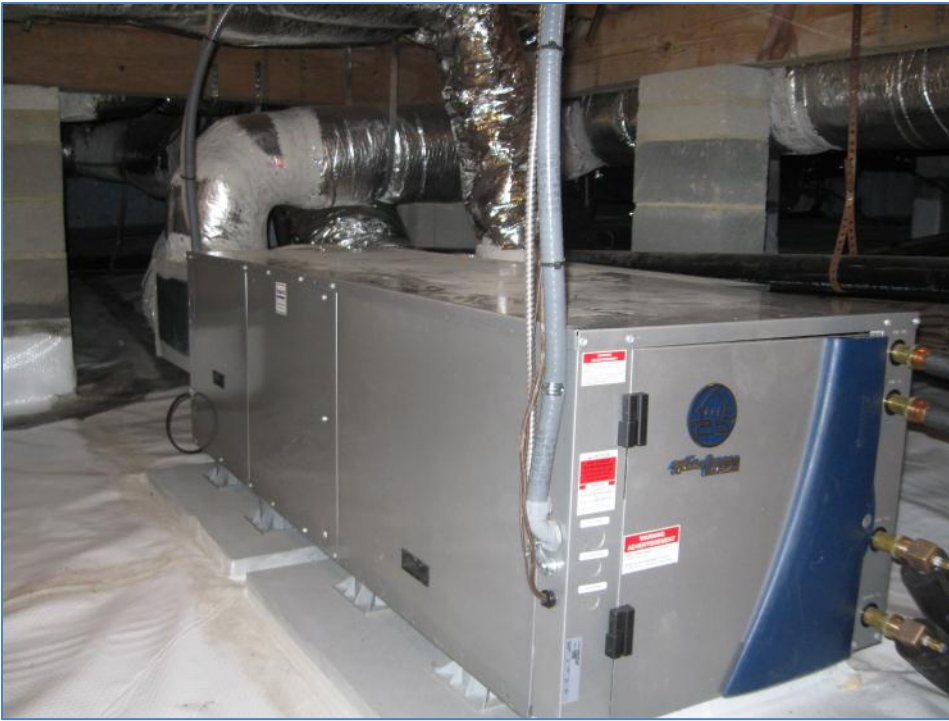
Photo: 31: Here's the completed Water Furnace Envision NDH-038 geothermal unit in our crawl space;
