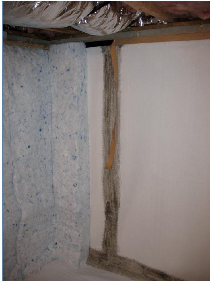
Photo: 36: Same image pulled back to view full length of foundation wall; note furring strip of wood over the insulation on the left;
